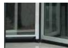
Side & Bottom Brushes to Prevent AC Loss
