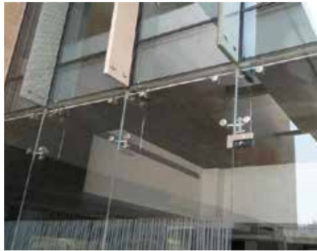
Ambience Tower, Gurgaon
